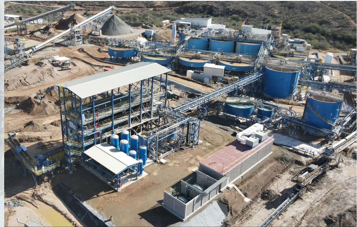
Santa Elena's Dual Circuit & New 3,000 tpd Filter Press
