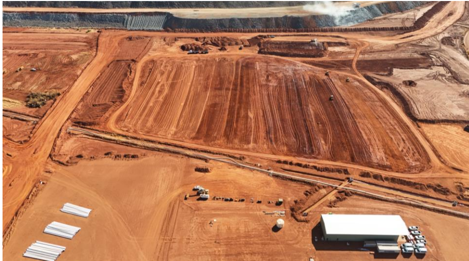
KEP Earthworks & Services
