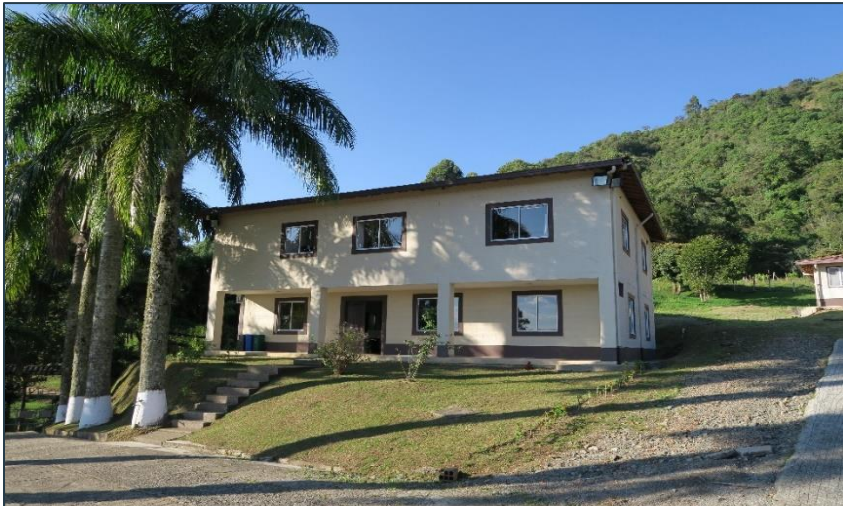
La Mina Office
