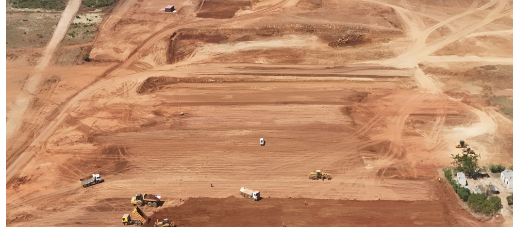
Process Plant earthworks CIL and Milling Areas progressing well.
