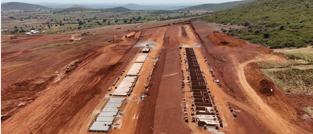
Terrace 4 & Terrace 5 – Senior Accommodation Buildings.
