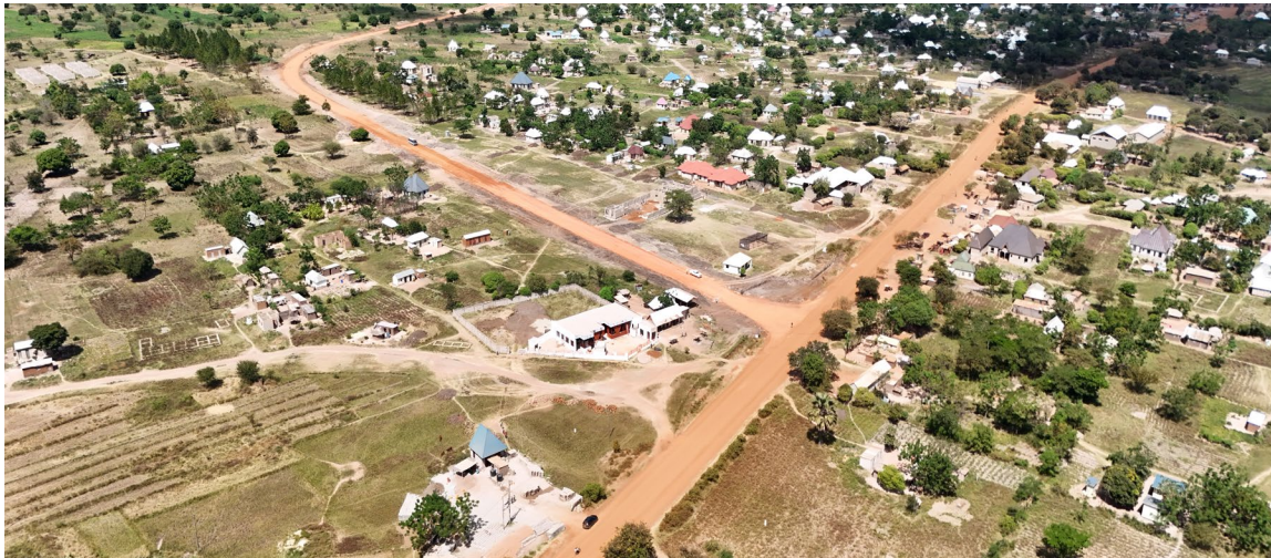
Ngoma Bypass Road – Roadworks on the Nyabila Bypass road Section
