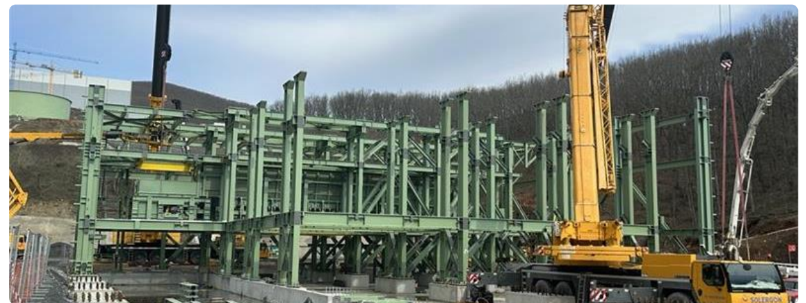
Filtered tailings building – close-up view
