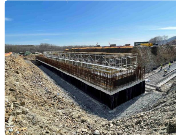
Coarse ore stockpile – reclaim feed tunnel
