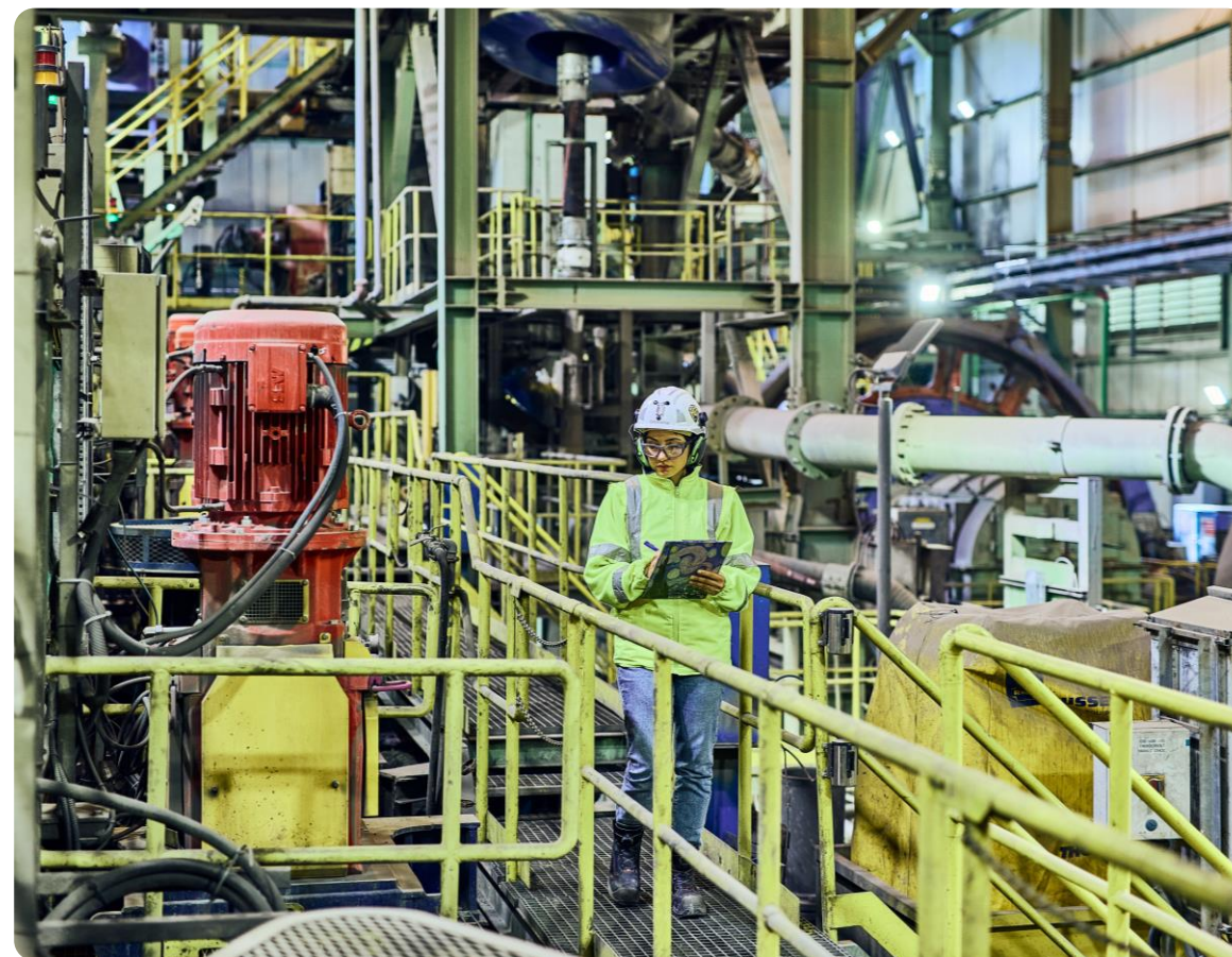
Process plant at Efemçukuru
