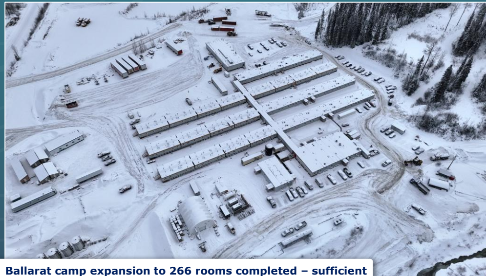
Ballarat camp expansion to 266 rooms completed – sufficient capacity for full construction manpower demand
