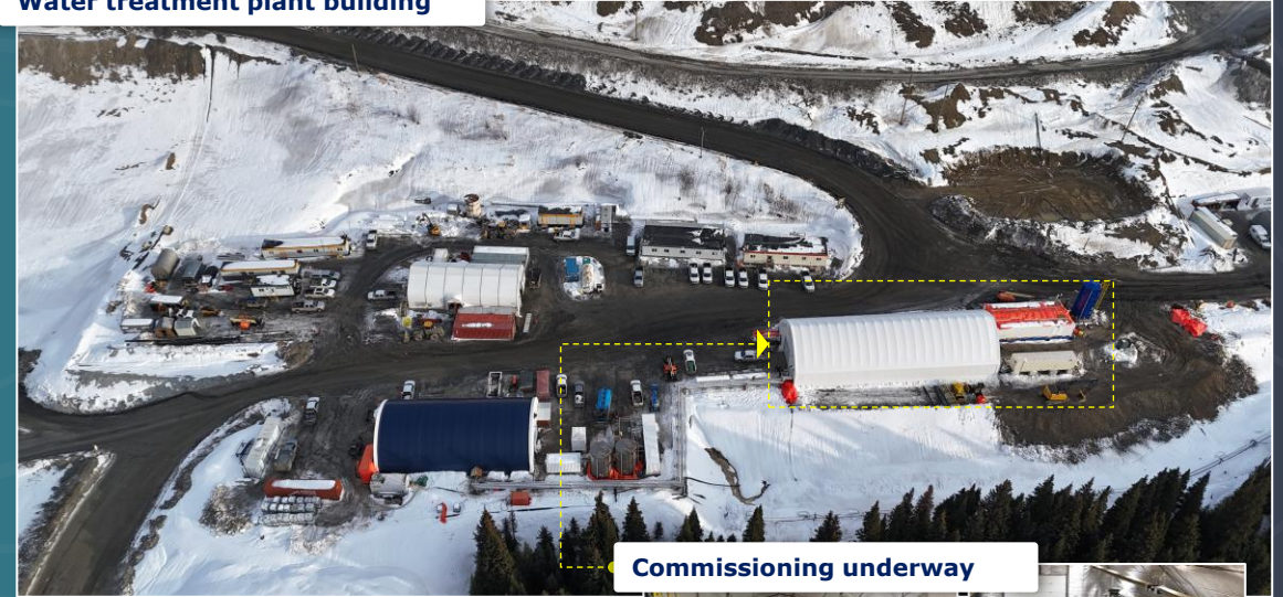
Water treatment plant building
