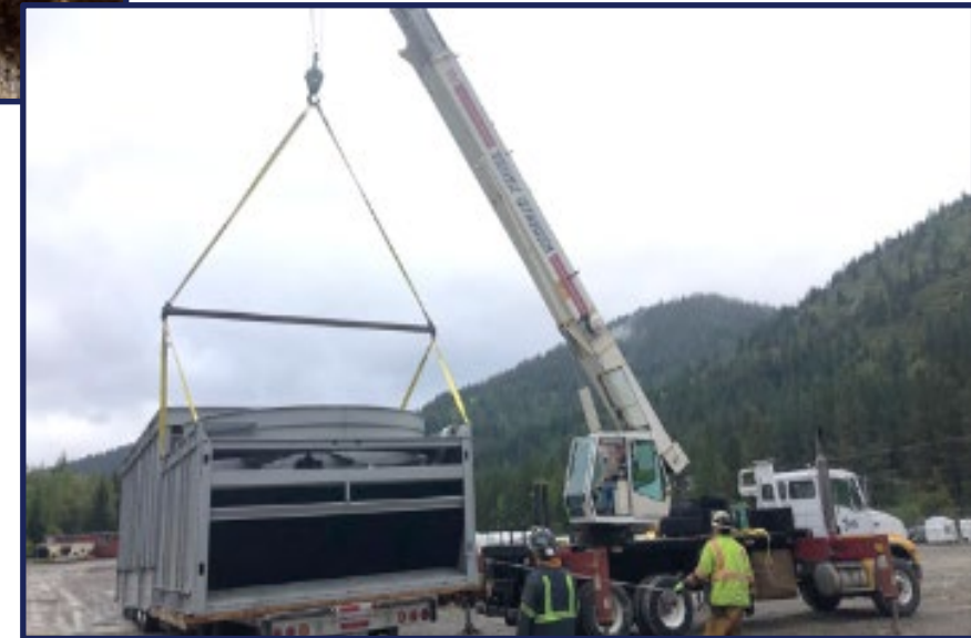
Surface Cooling Project
